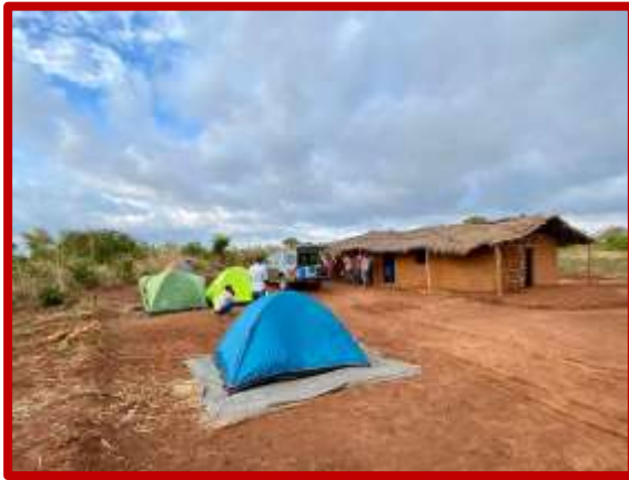
The newly erected prayer house in the Ribaué District
