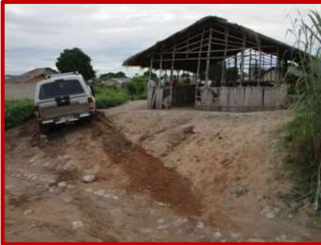
The structure that was destroyed by the first cyclone
